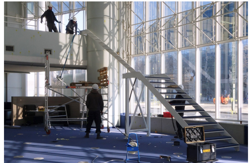
Figure 22 - Building dismantling services from Rotor DC. Image from rotordc.com
