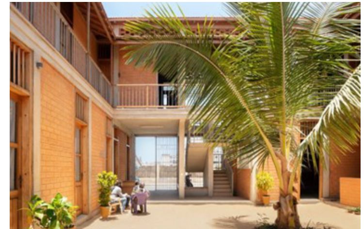
Figure 24 - Buildings constructed using ELEMENTERRE BTCs
